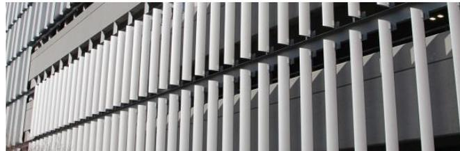
**Figure 18.** Movable vertical aluminium sun shading elements proposed to be applied on the east and west facades of the building [27]
