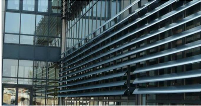
**Figure 17.** Movable horizontal aluminium sun shading elements proposed to be applied on the south facade of the building [26]
