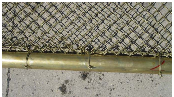
Figure 11. Double loop ties were placed every 20cm on the bottom net rim
