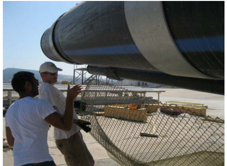
Figure 14. The net chamber being attached to the top pipe assembly
