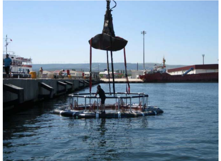
Figure 18. The cage being deployed into the water
