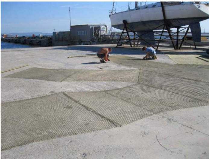
Figure 8. The bottom and top portions of the side panels were attached via helix coils.
