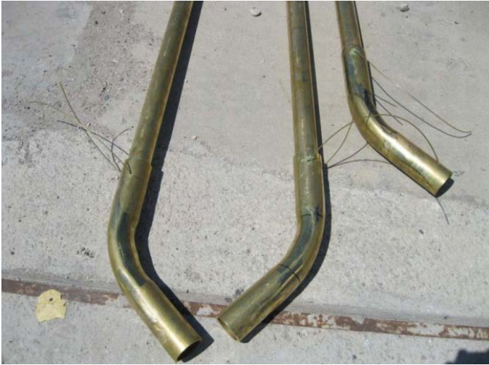
Figure 7. Each straight pipe length was first attached to a 45 degree elbow
