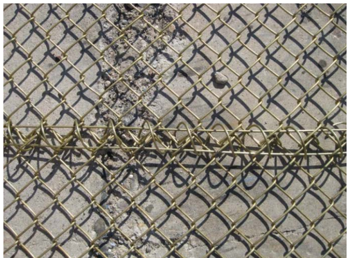
Figure 3. Helix coils were utilized to attach the two parts together
