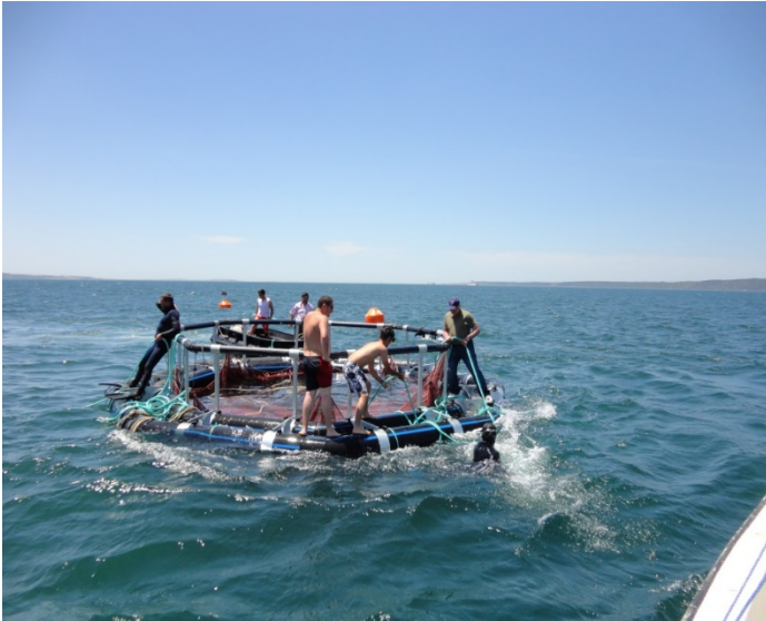
Figure 20. Securing the cage into the mooring grid
