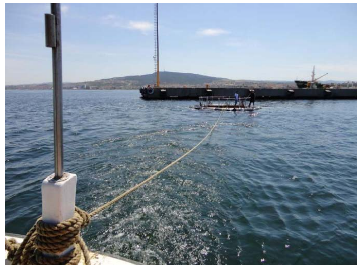
Figure 19. The cage was towed to the mooring site via a single line
