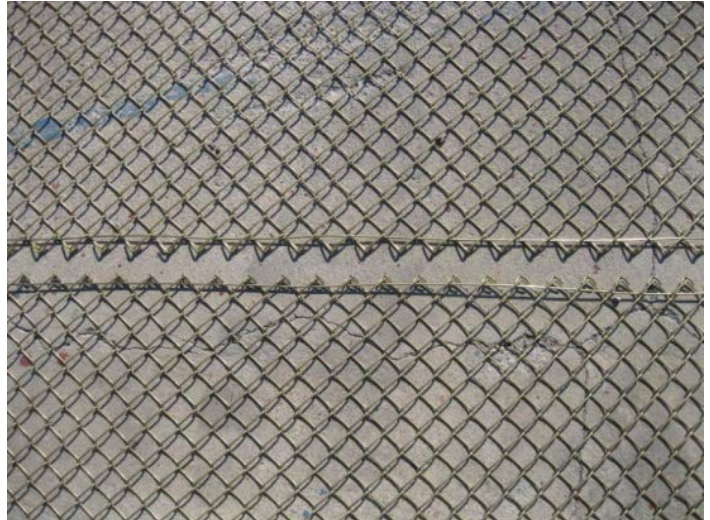
Figure 2. Straight wire was used to outline all edges of the mesh
