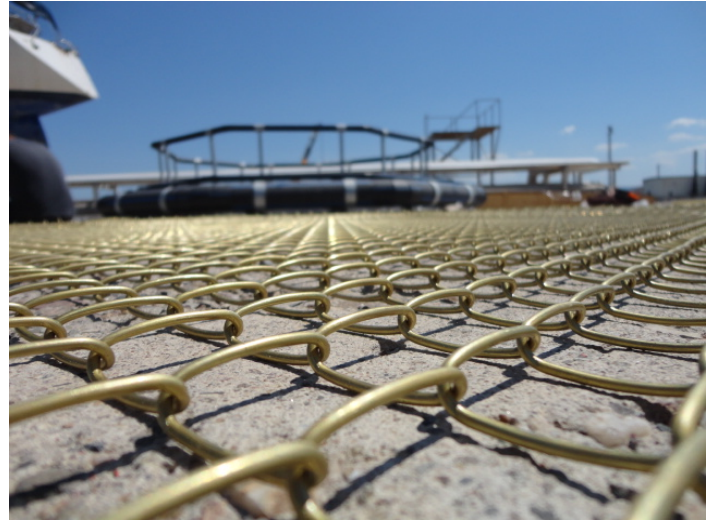
Figure 6. Copper alloy chain link mesh panel laid out near the cage frame
