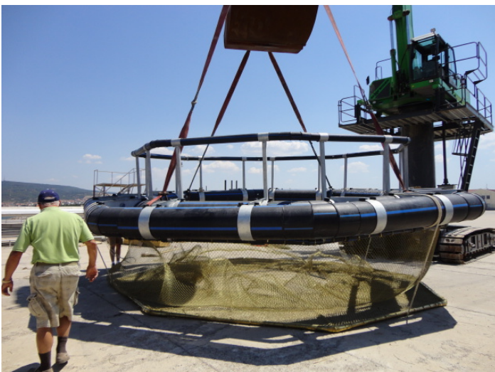
Figure 17. Bridle lines placed under the cage for lowering the system
