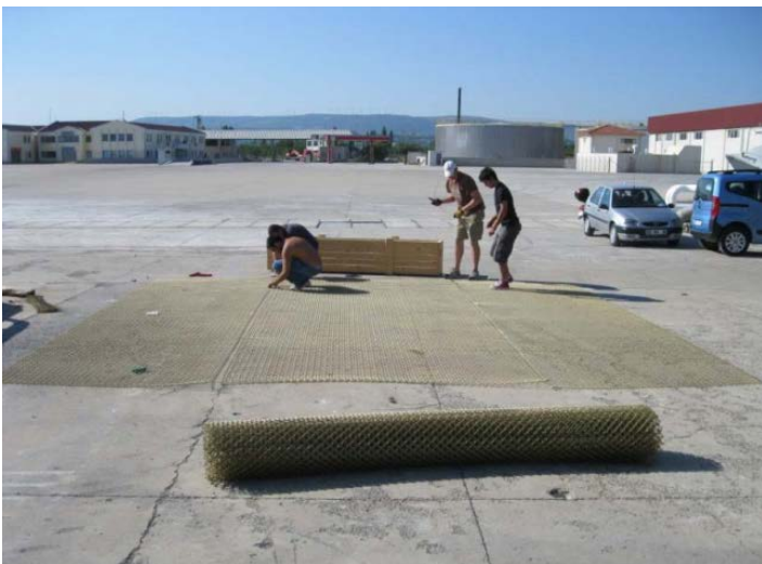
Figure 1. Two lengths of 1.75 m mesh were positioned on both sides of the 2.5 m mesh to form the bottom net panel
