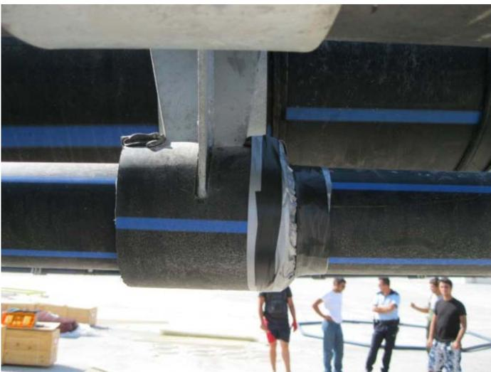
**Figure 13.** Insulating tape covering exposed metal to prevent galvanic corrosion.
