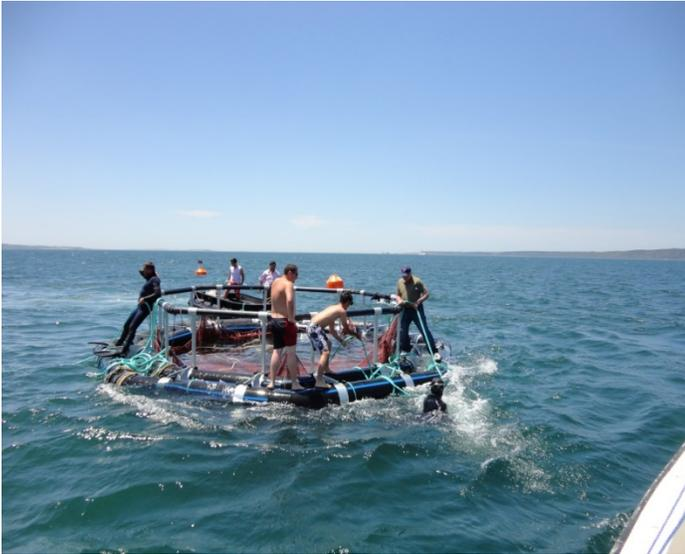
**Figure 20.** Securing the cage into the mooring grid
