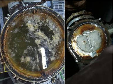
Fig. 5. Seawater Inlet filters after mucilage effects (DTO, 2021)
